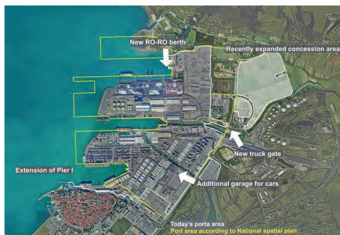
Figure 23 - Infrastructural improvements in the Port of Koper - Source: Luka Koper's own elaboration
